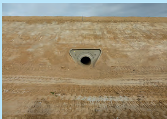
Terrassement routier. © Cerema
